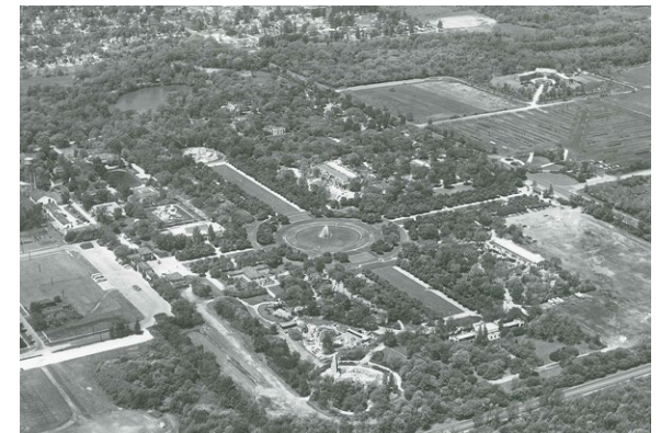
North, South, and East Malls
